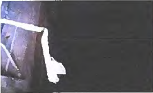
Photo 10-3 Loose/ unterminated wire
