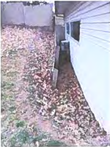
Photo 2-1 Retaining wall is leaning and should be monitored. Suggest having a contractor evaluate it.
