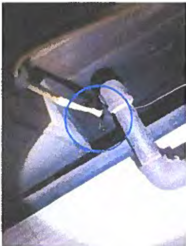
Photo 4-1 Recommend filling with foam
