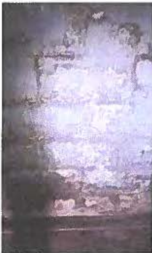
Photo 8-3 Efflorescence on the front middle basement wall
