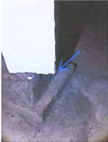
Photo 2-1 Post has twisted and moved about 1/3 off the pier.
