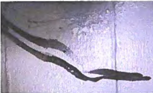
Photo 10-5 Loose/unterminated wire
